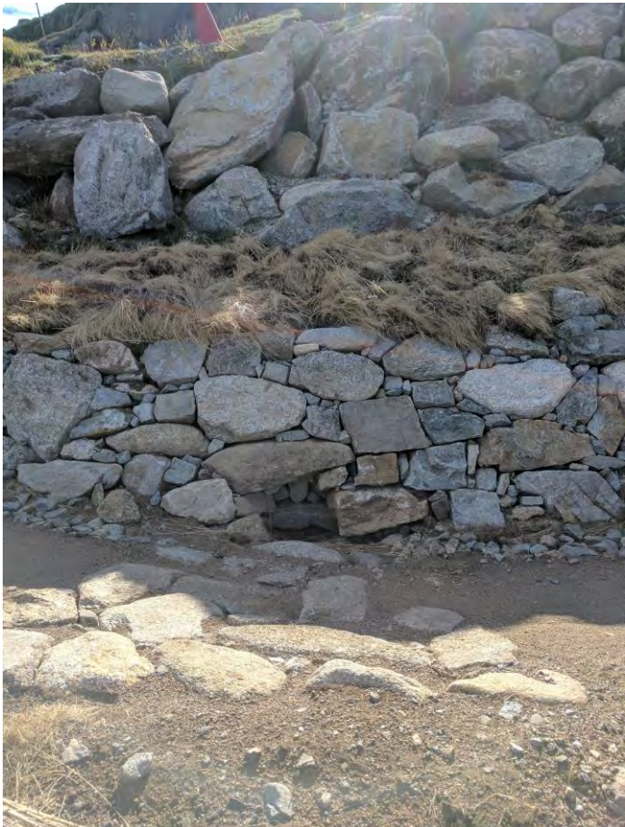
Figure 9: Example of drainage incorporated into the corners
