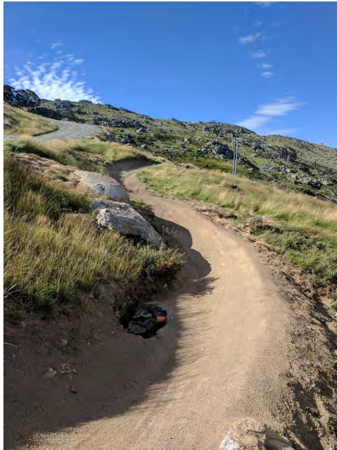
Figure 10: Example of drainage incorporated into the corners
